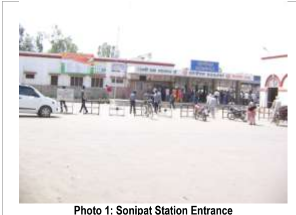
Photo 1: Sonipat Station Entrance
