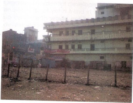
View of Part A of the site
